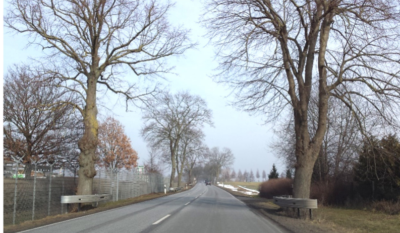
Fig. 2 Example for a short barrier construction to protect a single obstacle next to the road
