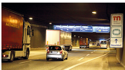
Heavily trafficked road tunnel (Photo: BMVI / René Legrand)
