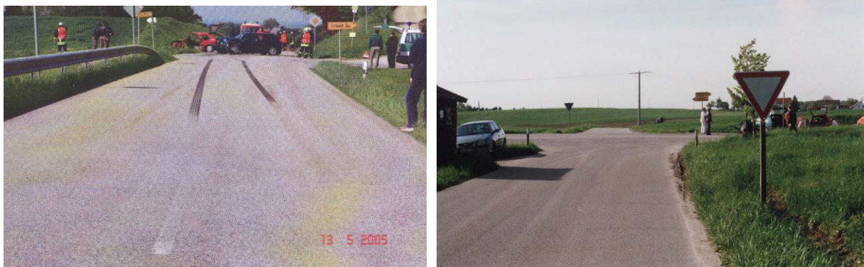
Figure 10: Case 8 – Road lay-out at scene
