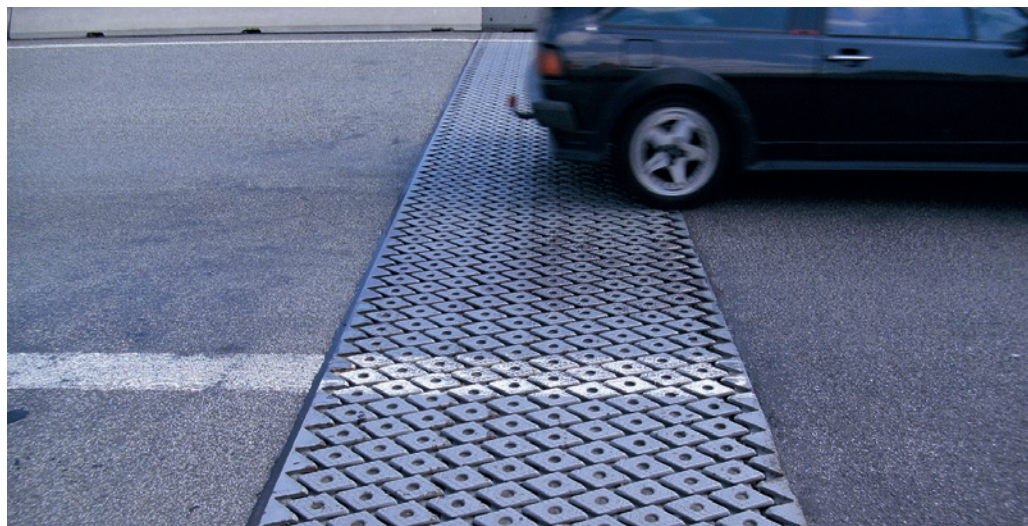
Expansion joint in steel blade construction with noise mitigation
