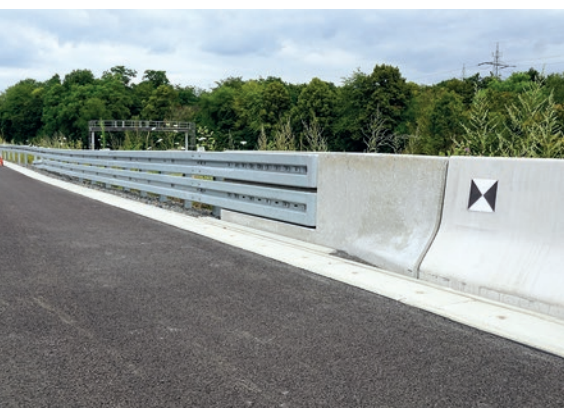
Transitions to connect different safety barriers
