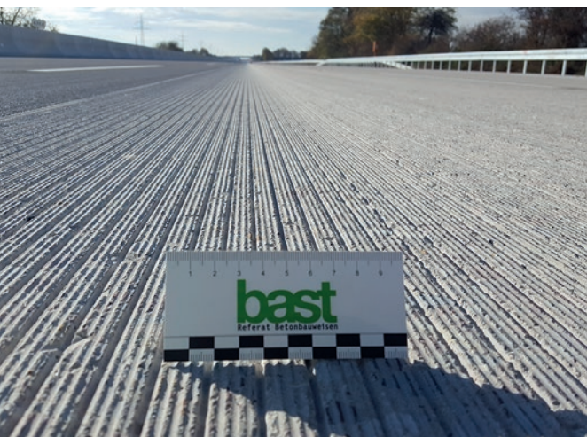
Road surface texture grinding: typ S+ 2.4/2.2 – 2.4/18
